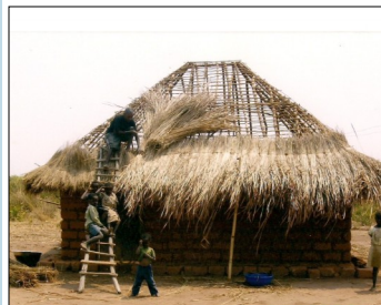
New Thatch for the Roof
